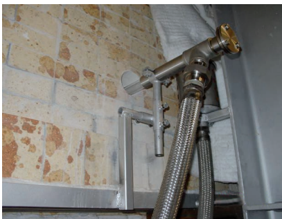
STG Furnace pressure probe installed
